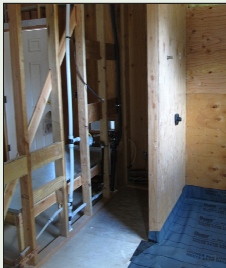
Site for Swamp Cooler Entry Point
