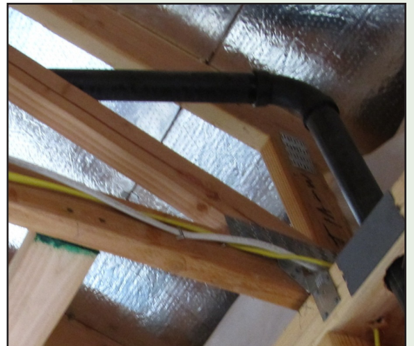
Raised-Heel Roof Truss
