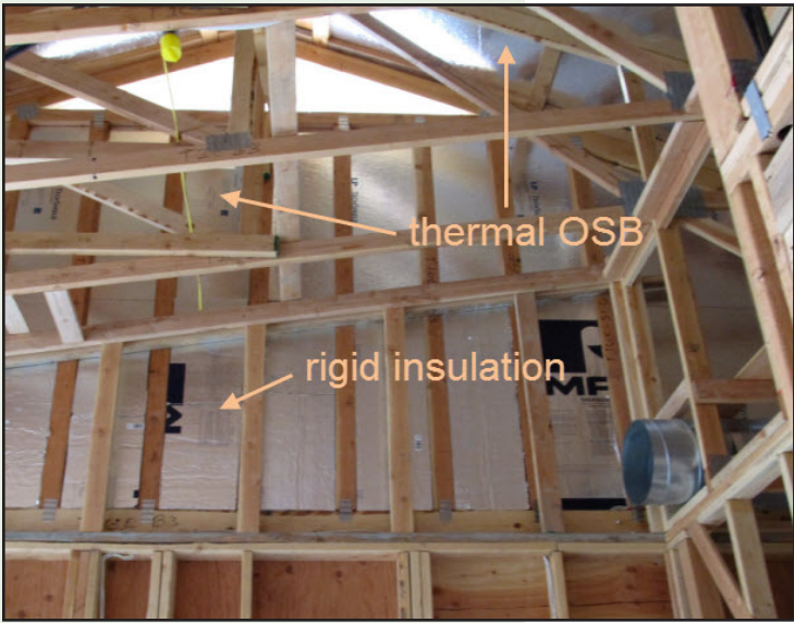
Rigid Insulation and Thermostat OSB on High Walls and Attic Ceiling
