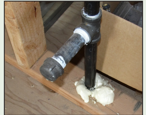
Hard-Setting Foam to Seal Pipe Hole
